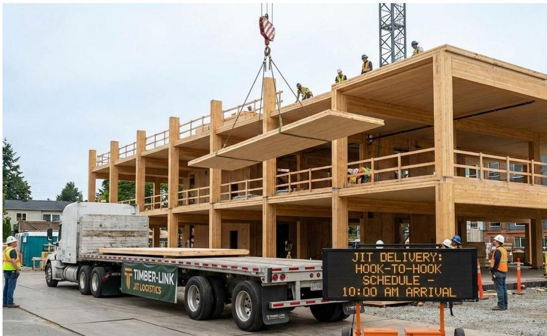
Figure 2.1. JIT logistical model on a construction site
