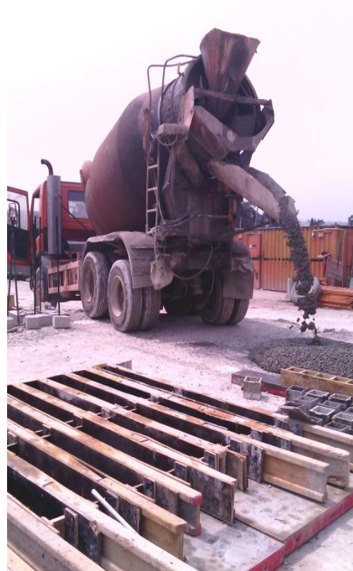
Fig. 2 Casting of concrete to the beams and cubes
